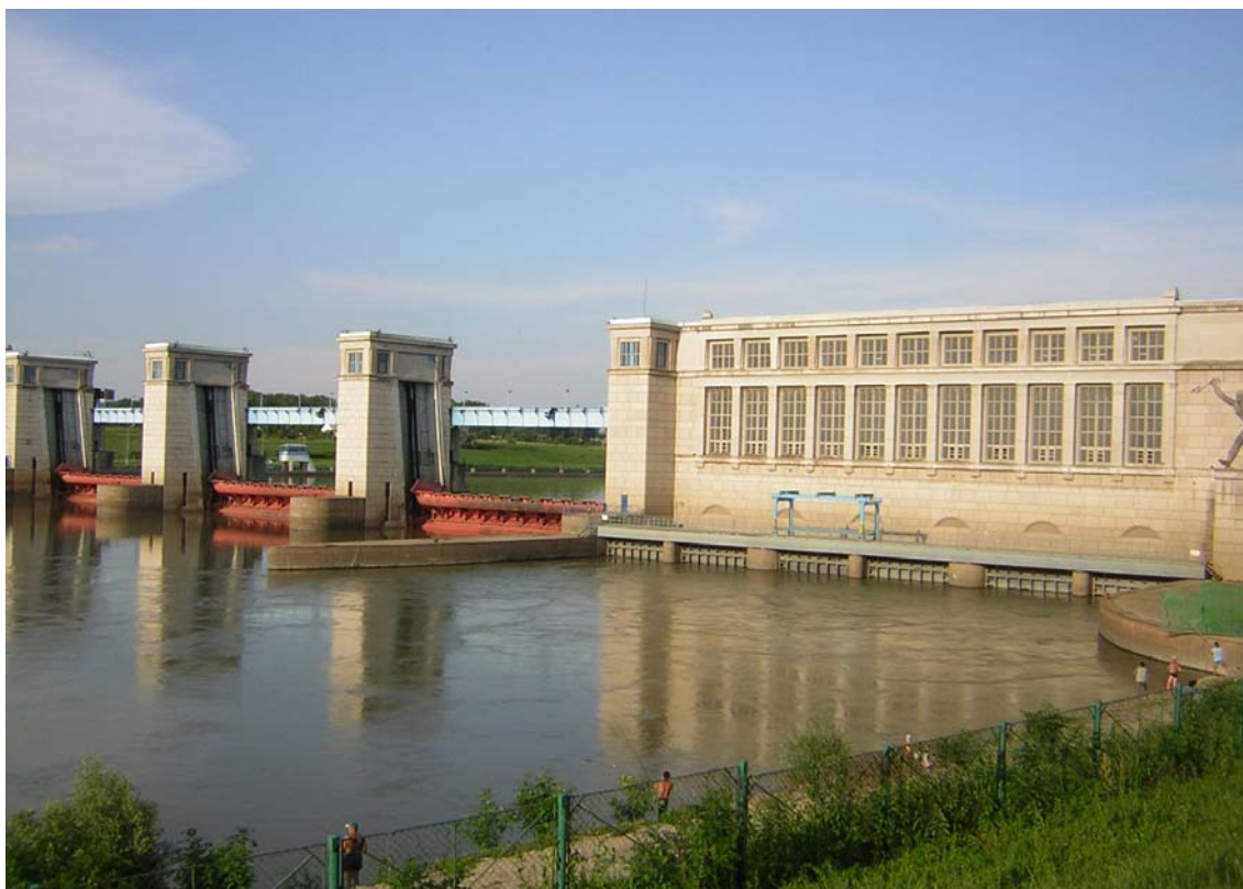
The Tysa - hydropower plant - photograph by Tomasz Walczykiewicz
